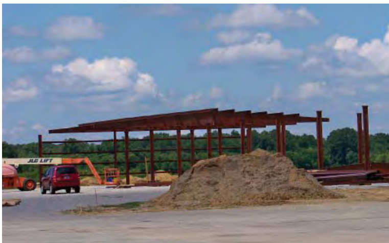
New T-hangar construction
