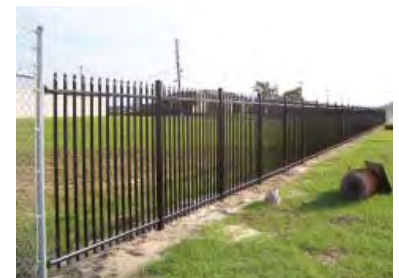
Security fence construction
