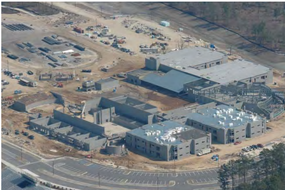
Construction of the new Colleton County High School in progress
