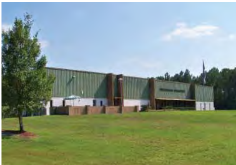
RBC Linear building acquired by Paper Converters
